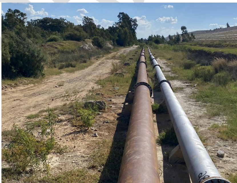
FIGURE 5-1: EXAMPLE OF PIPELINE ON CONCRETE PLINTHS WITH ADJACENT ACCESS ROAD
